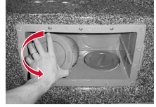
Turn Filter Counter-clockwise to Remove
